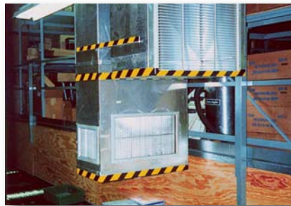
Striped 3M™ Vinyl Tape 5702 calls attention to protruding equipment and steps. 132
